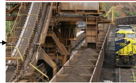
15 km existing road to rail terminal.
